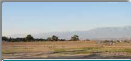
Oak Street Stormwater Retention Basin
